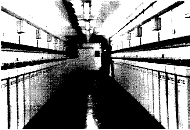
Fig. 5. One of the battery rooms at BEWAG plant in Berlin–Steglitz.
